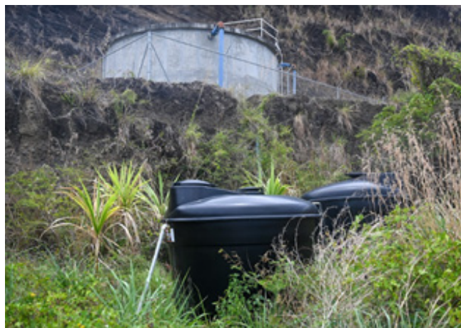
Water storage tank and associated reservoirs constructed under the project.
