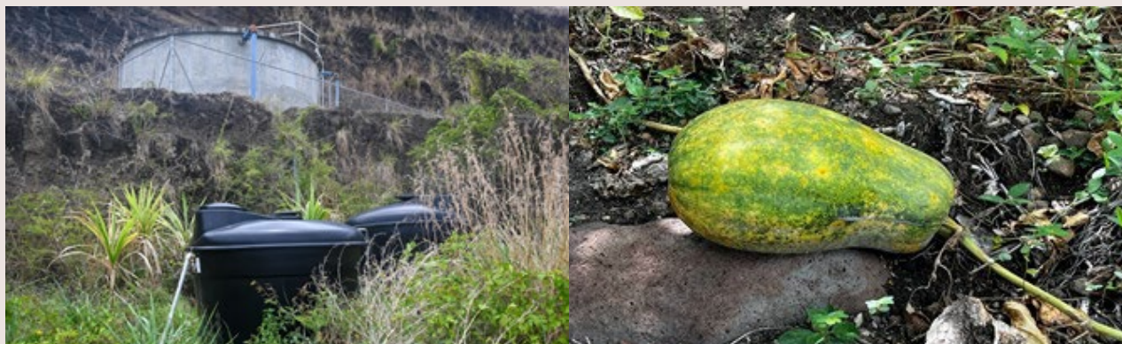
On left, water tanks constructed under the project; on right, a vegetable grown using water provided under the project.
