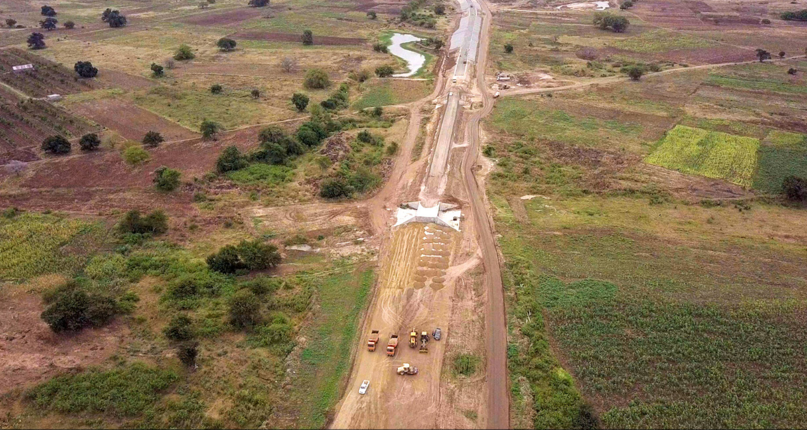
Roads and Bridges Management and Maintenance Project in Chókwè, Mozambique.
