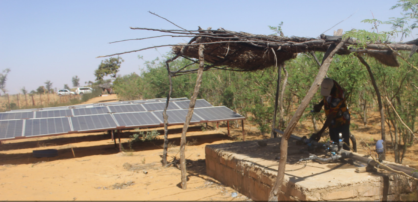
A solar-powered drip irrigation installed under the Niger Irrigation Program. Photo: Amel El Abed/CIFF
