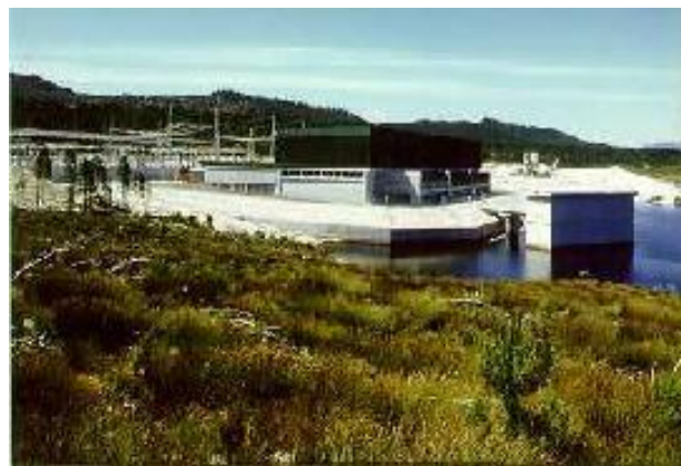
Palmiet Pumped Storage Installed capacity: 400MW (for 28 hrs)
