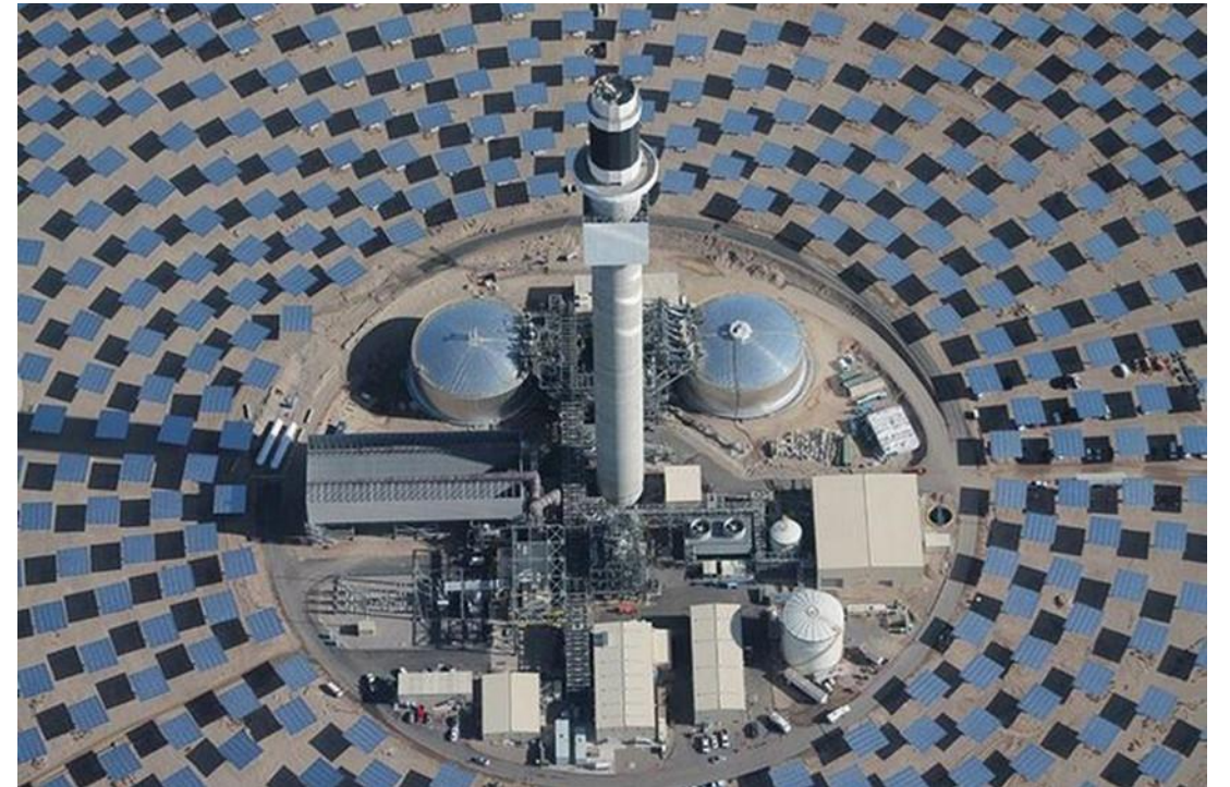
Crescent Dunes Solar Tower, NV (110 MW e with 10 hrs storage (1.1 GWh e ))
