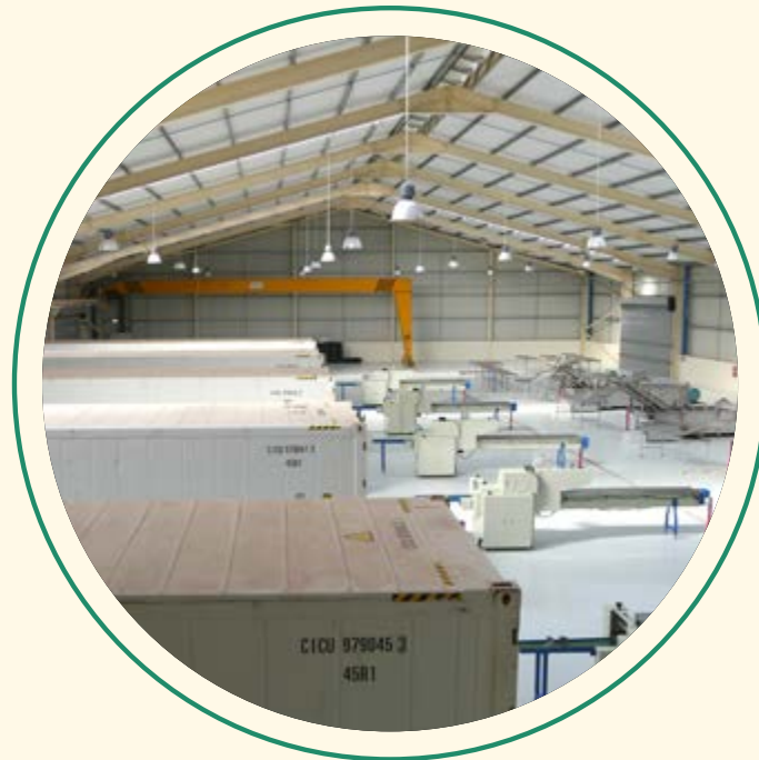
Processing Center for Vegetables and Fruits - CEPHOL (Baixo Limpopo Irrigation Scheme, Gaza) - BLICRP
