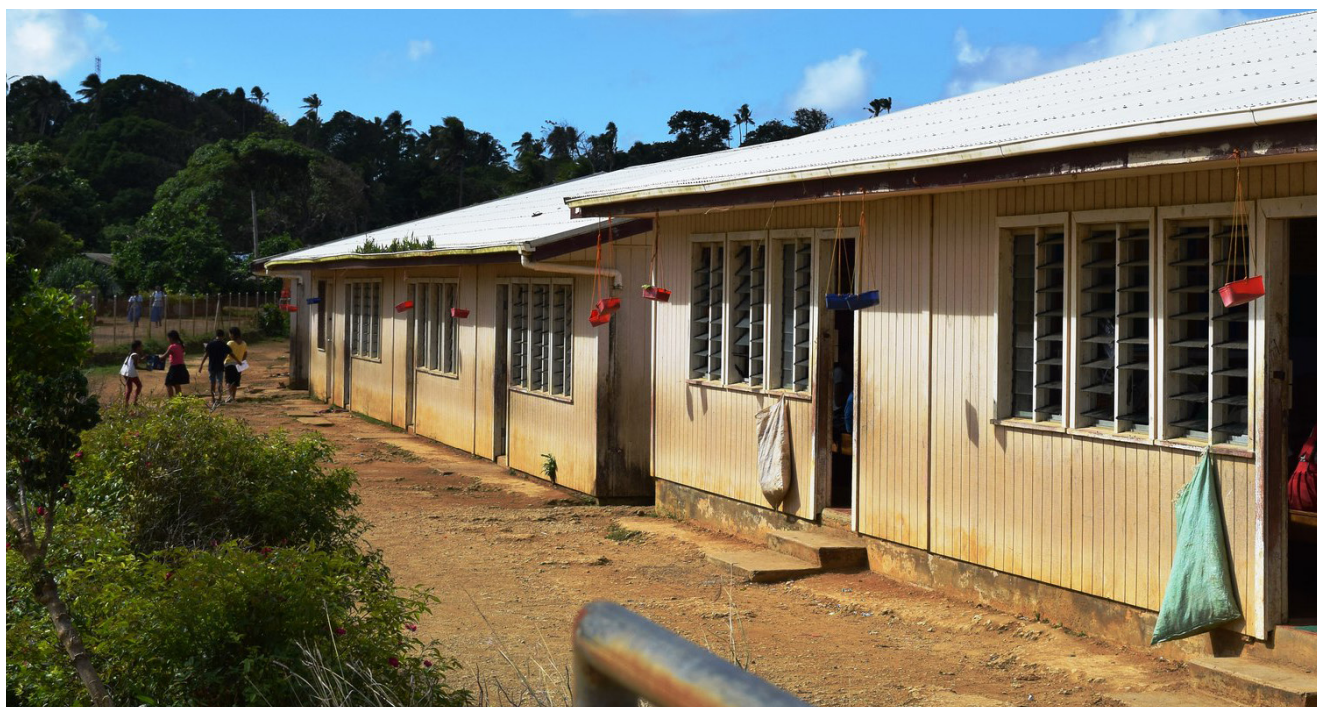
Climate-proofing of a school in Tonga
