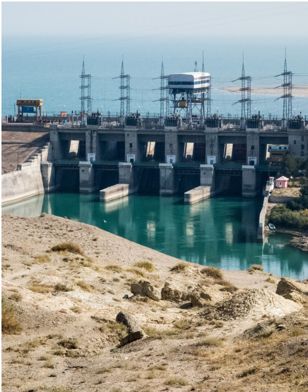
Safeguarding critical dam infrastructure in Tajikistan
