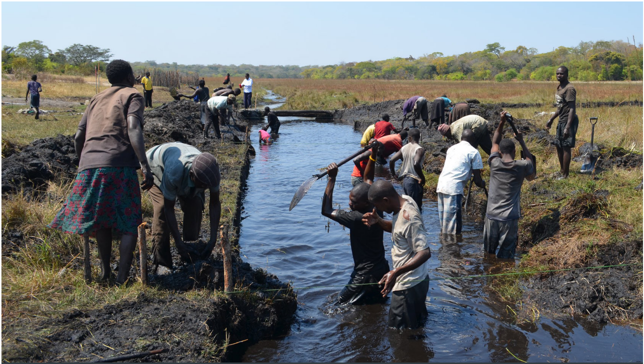
Canal digging in Zambia
