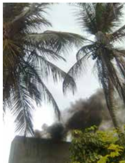
Black smoke emitted from a small powerhouse
