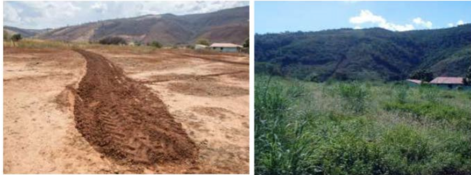
Result of the implementation of a system of contour lines: before (left) and after (right)
